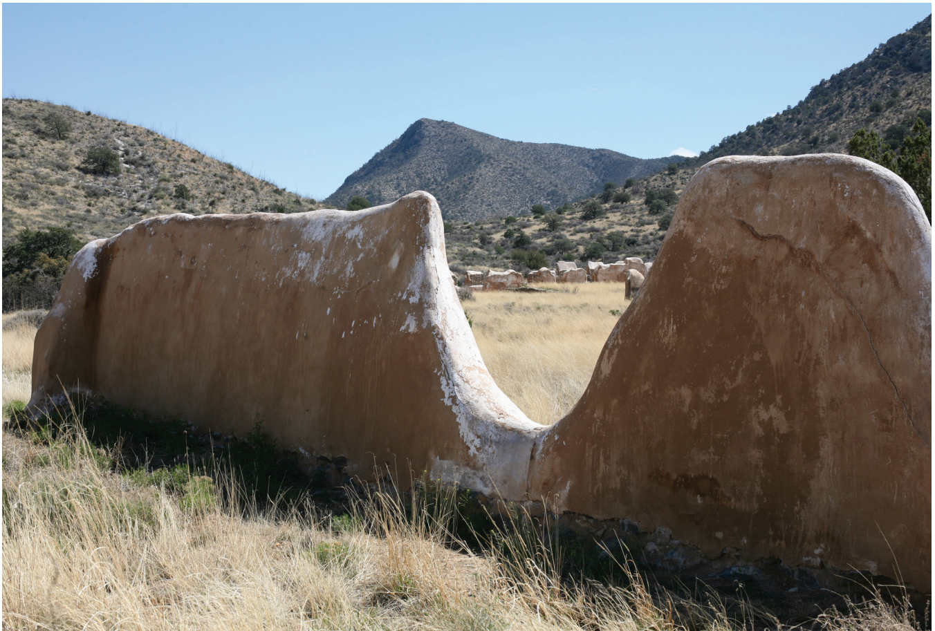
Figure 3. Lime-plaster encapsulated ruins of the historic corral wall at Fort Bowie NHS. Rangers colored the plaster to match the local soil; the lime coating is beginning to wear away exposing the uncolored plaster. View looking southeast. Photograph by R.L. Pinto, 2017.
