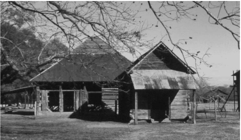
Figure 4. Carpenter's Shop and Mule Barn, Oakland Plantation. National Park Service photo.
