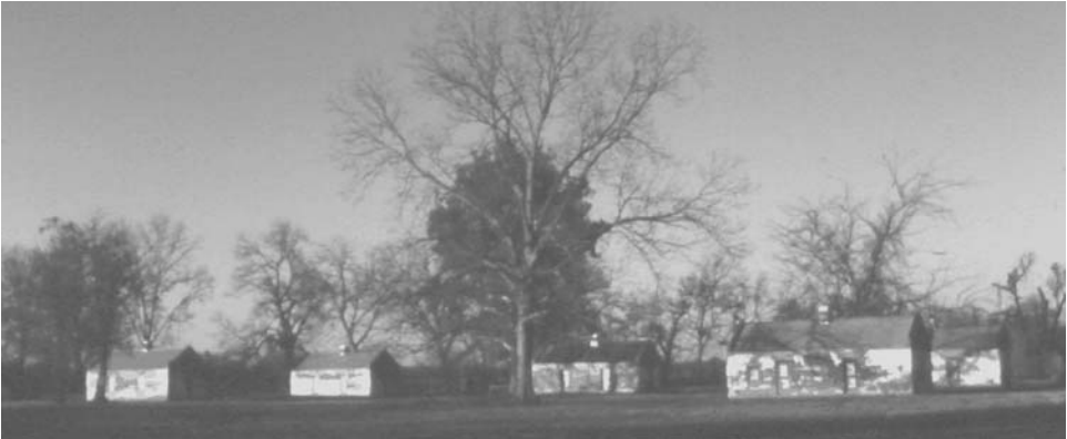
Figure 6. Brick slave quarters, later used as housing for tenant farmers, Magnolia Plantation. National Park Service photo.
