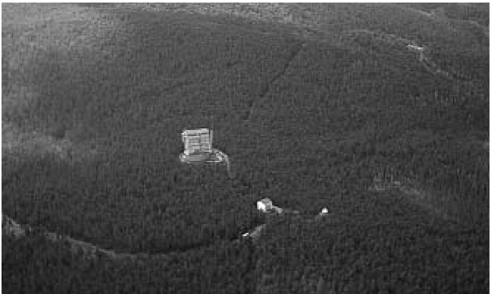
Figure 1. An aerial view of the telescope complex on Mount Graham, July 1999. Photo by Rick Teachout courtesy of Large Binocular Telescope Project.
