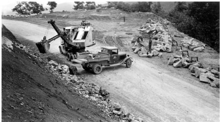
Stone guardrail under construction on Skyline Drive, early 1930s. National Park Service photo, courtesy of Shenandoah National Park collections.
