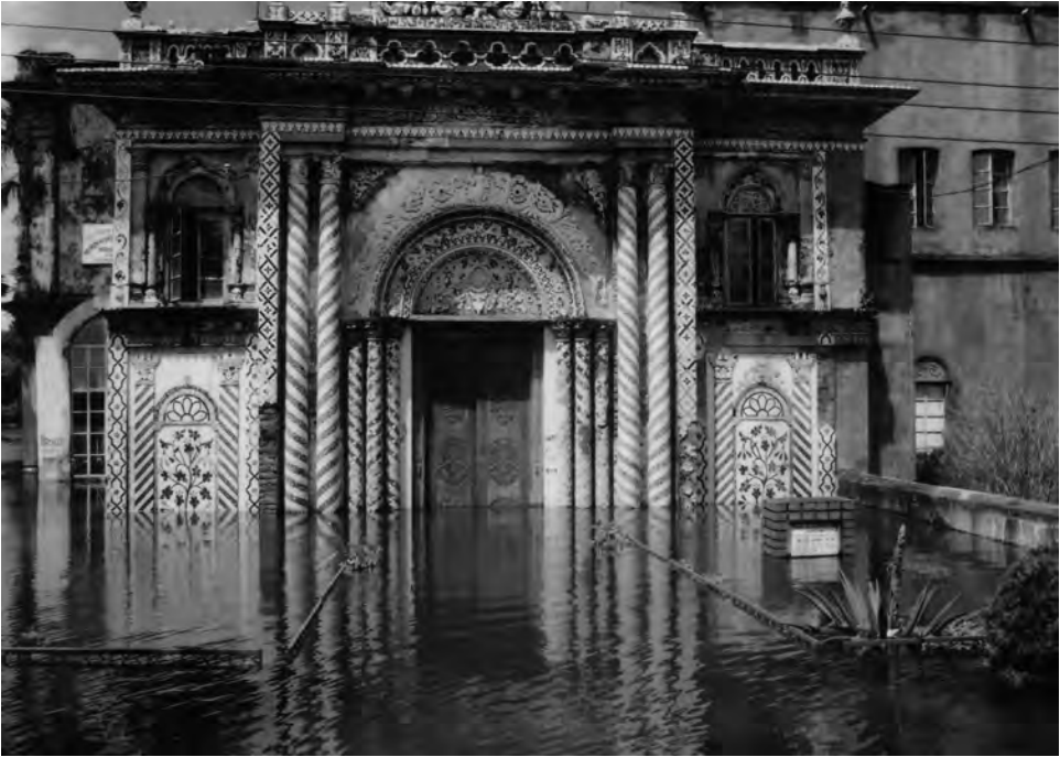
Figure 8. A flooded historic building in Sonargaon, Bangladesh. Photo courtesy of World Monuments Fund.
