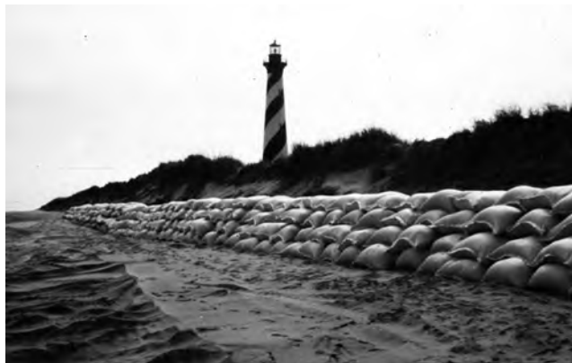
Figure 4. Sandbag seawall in front of Cape Hatteras Lighthouse, taken shortly after the seawall was constructed in 1971. The seawall was destroyed by wave action soon thereafter. Source: USGS 2007b. R. Dolan photo courtesy of U.S. Geological Survey.
