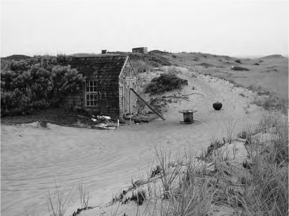
Figure 3 The Tasha Shack, in the Dune Shacks of the Peaked Hill Bars Historic District, Cape Cod, Massachusetts. Photo courtesy of Chuck Smythe.
