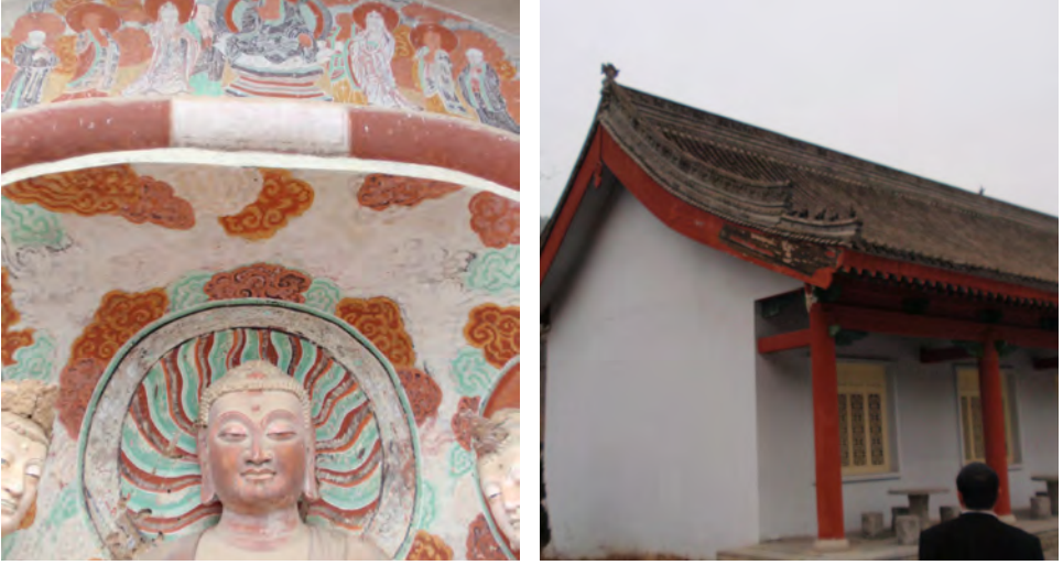
Figure 4. Maintenance contrast: Paints in the grotto caves (left) are still vibrant centuries after they were applied; meanwhile, paint near the roof of a much newer support building (right) is already giving way to the elements. Photo courtesy of NPS/Tim Harvey.
