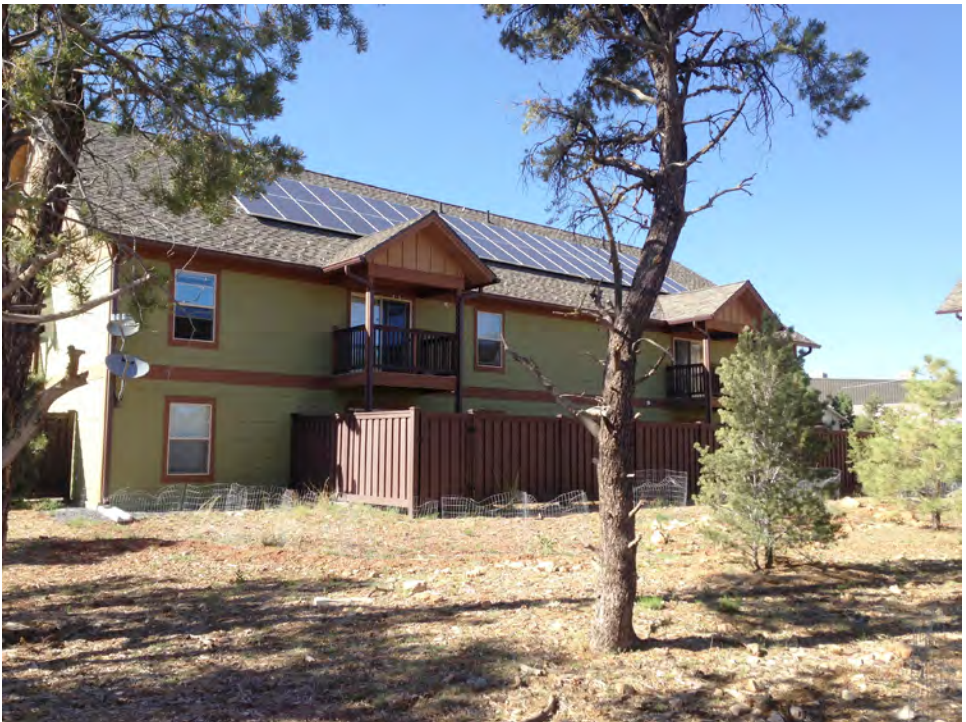
Figure 5. Grand Canyon National Park’s Paiute Apartments received a LEED Platinum rating for their sustainability features. NPS photo.
