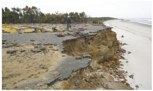
Figure 4. Erosion at the Sandy Hook Nike Missile Launch site caused by Hurricane Sandy storm surge.
