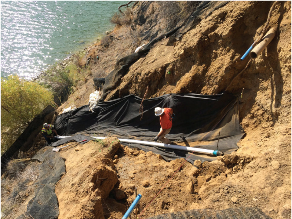
Figure 3. An EBRPD construction crew repairs a storm-damaged water line caused by a landslide at Del Valle Regional Park (EBRPD).
