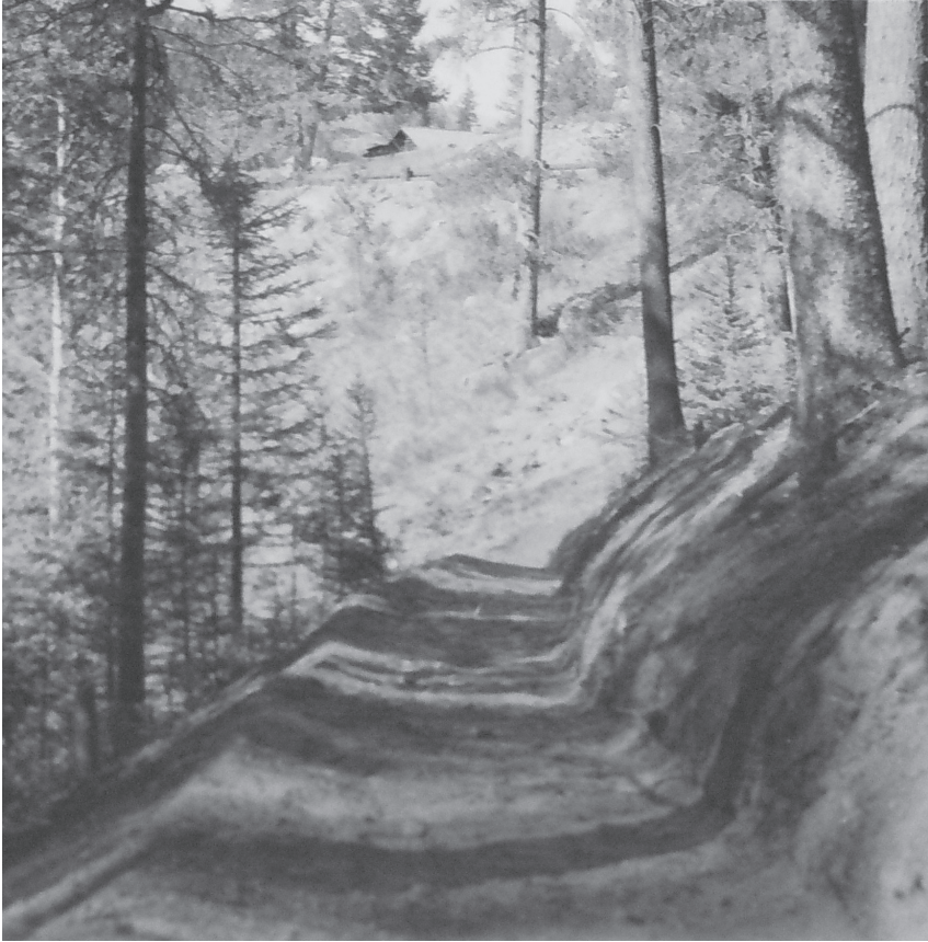
Figure 5. Completed New Howard Eaton Trail. By the end of the 1930s, the HET was wider, smoothly graded, and dead trees and other debris had been removed from the area on either side of the trail. Photograph titled "Howard Eaton Trail, completed along side hill. Tower Falls, 7-27-36, Jacobson," courtesy of Yellowstone Heritage and Research Center Museum, YELL 192993-1159.
