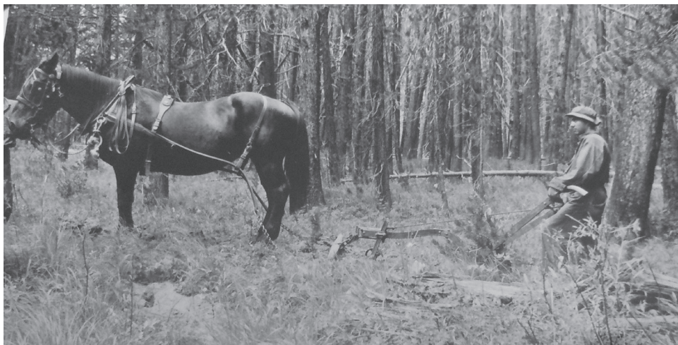
Figure 3. Building the second Howard Eaton Trail. Photograph titled “Plowing out ditch along trail at Arnica Cr. (Lake), 7-29-36, Jacobson,” courtesy of Yellowstone Heritage and Research Center Museum, YELL 192993-1161.
