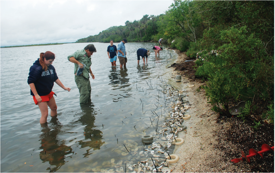
Figure 1. Workers install oyster shell mats as part of the living shoreline project in Mosquito Lagoon at Canaveral National Seashore. M. Schwadron/National Park Service photo.
