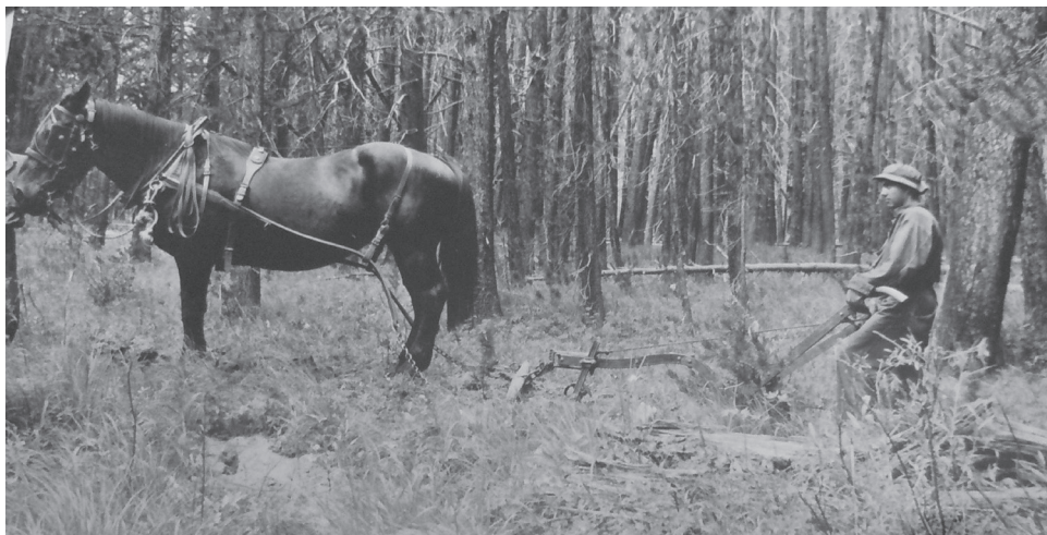
Figure 3. Building the second Howard Eaton Trail. Photograph titled “Plowing out ditch along trail at Arnica Cr. (Lake), 7-29-36, Jacobson,” courtesy of Yellowstone Heritage and Research Center Museum, YELL 192993-1161.
