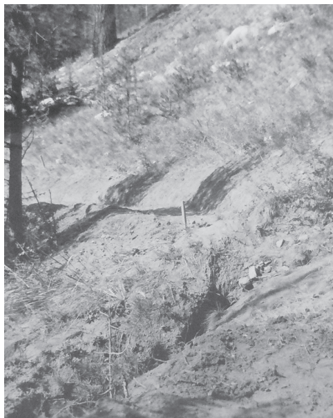
Figure 4. Condition of the Howard Eaton Trail prior to reconstruction. Photograph titled “Side hill gully before rip-rapping with rock, Tower Falls, 7-27-36, Jacobson,” courtesy of Yellowstone Heritage and Research Center, YELL 192993-1158.
